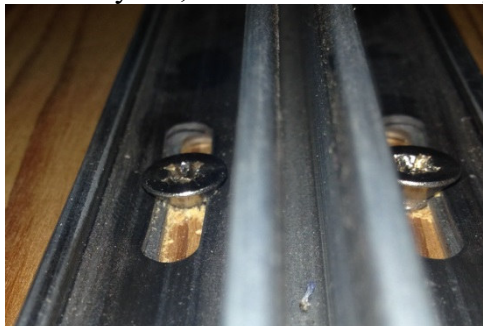
Figure 1. Countersunk head screws fixing the inox profile with limited movement capacity
